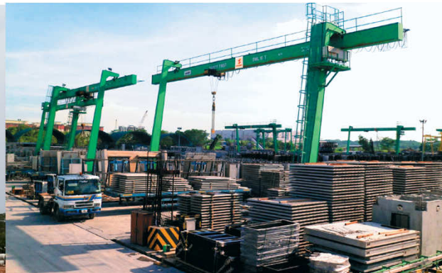
Precast Yard in Singapore
